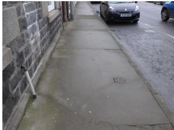
Shore Street footway
